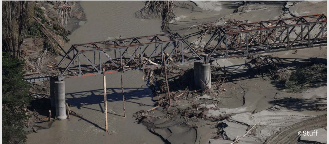
Figure 1. Top: forestry debris piled up on a railway bridge over the River Esk. Note the debris attached to the top of the bridge shows the magnitude of exceedance of design standards. Bottom: extensive silt deposition on the lower reaches of rivers devastated farmland and infrastructure, recovery will take years
