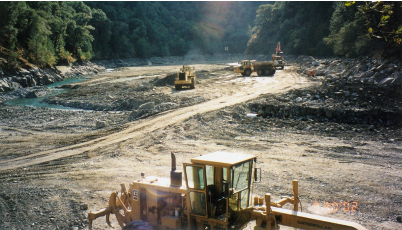
Sediment removal operation at PCWA's Ralston Afterbay facility. © PCWA
