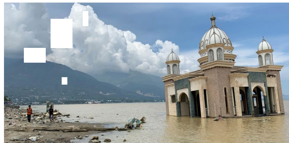
Masjid Apung Mosque in Palu, Indonesia, currently subjected to inundation due to coastal settlement from the 2018 Sulawesi Earthquake and Tsunami. (Source: EEFIT and T.Rossetto)
