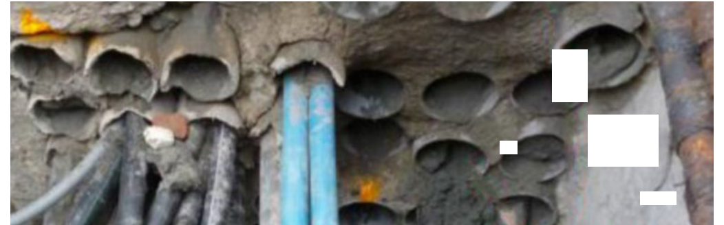
Figure B: Liquefaction manifestation observed inside a telecommunication Utility hole. (Photo courtesy of Rob Ruiter, Chorus Ltd.)
