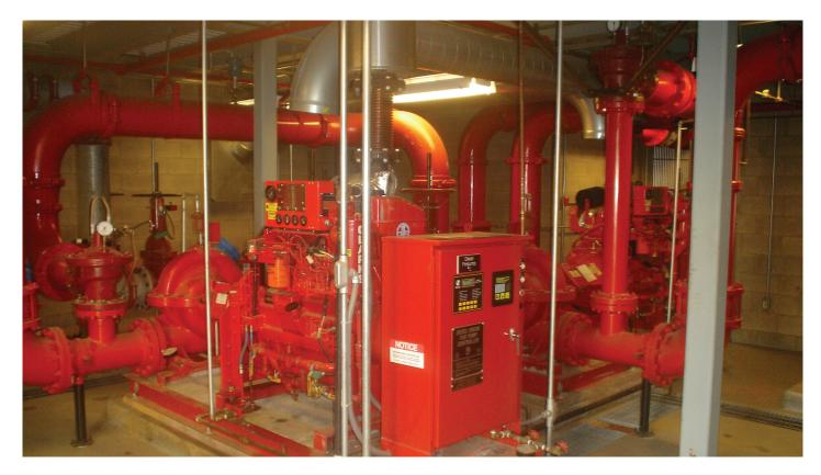
Pictures showing a fire pump and a hose monster after a fire pump flow test. The underground water main supplying the pump had not been properly flushed prior to installing the fire pump.
